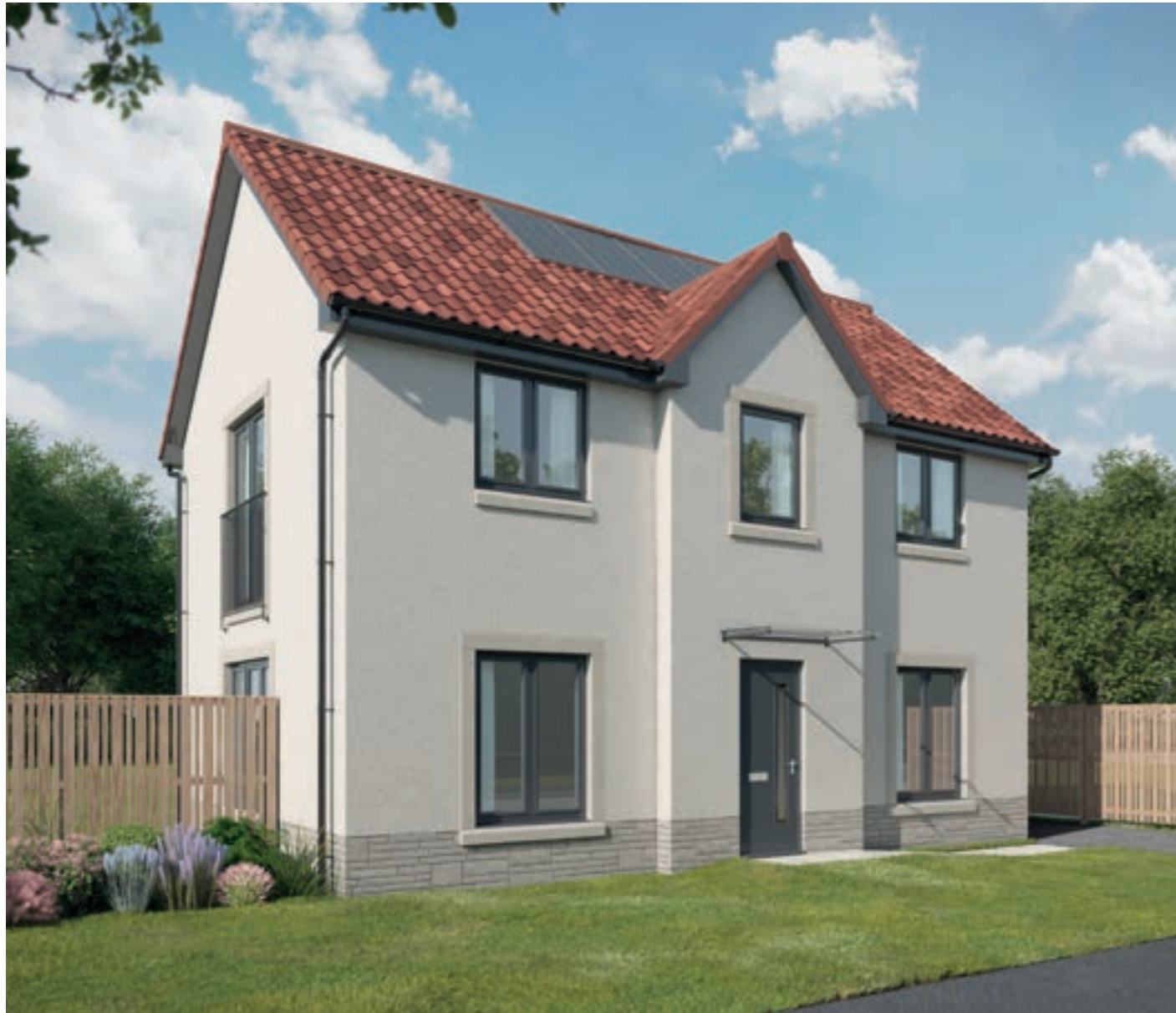
Please note Photo Voltaic (solar) panels shown above are indicative only. The location and number of panels are dependent on plot orientation. Please see Sales Advisor for details.
