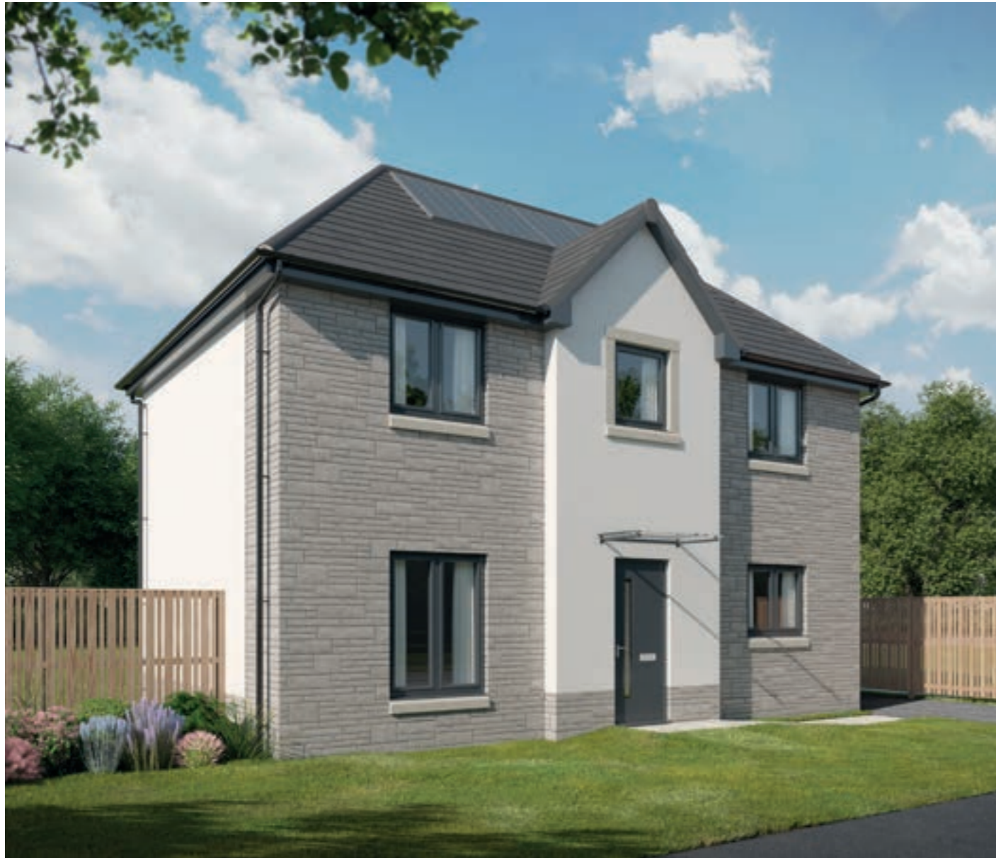
Please note Photo Voltaic (solar) panels shown above are indicative only. The location and number of panels are dependent on plot orientation. Please see Sales Advisor for details.
